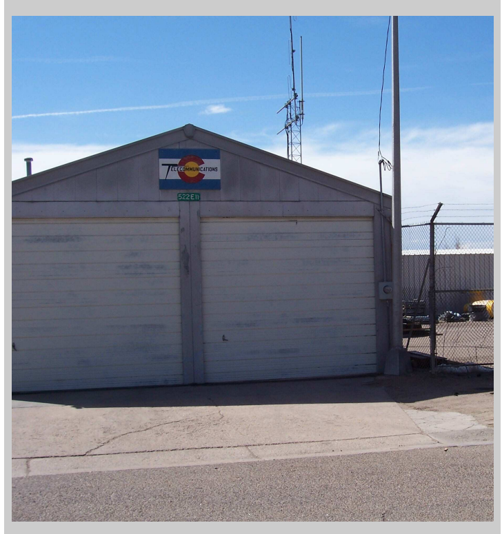
Typical maintenance facility, with potential hazardous material storage in yard.
