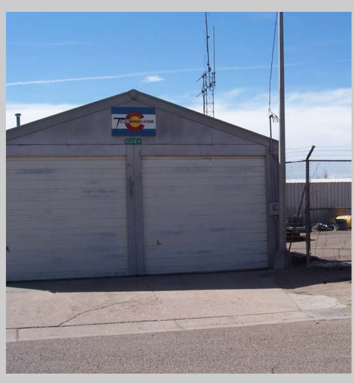
Typical maintenance facility, with potential hazardous material storage in yard.
